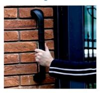
A grab bar at an entrance provides support and makes it safer and easier to open an entrance door. The key feature of this plastic grab bar shown in the picture is that it is rust proof and in winter, will not get as cold as a metal grab bar. Weight capacity of a recommended grab bar in general is 250 pounds and above.
