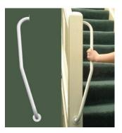
Specially designed grab bars can be installed on the walls alongside the stairs. The key feature of the grab bar shown is that its curved design allows for continuous support around the corner of the stairs.
