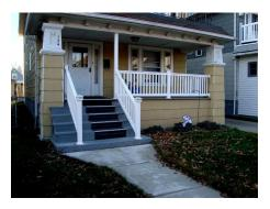
Hand railings on both sides of the stairs will provide support for safely climbing and descending the stairs. Vinyl railings have advantages over wooden or metallic railings in terms of durability, maintenance costs, corrosion, resistance to mold, and decay.
